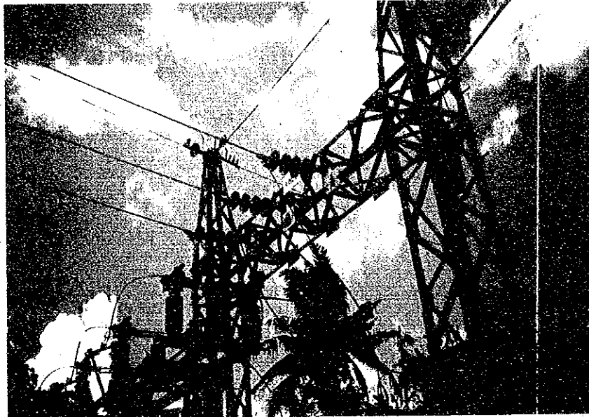
Photo 2-1 Airai Substation was built under the fiscal 1984/1985 Japanese Grant Aid Project.
