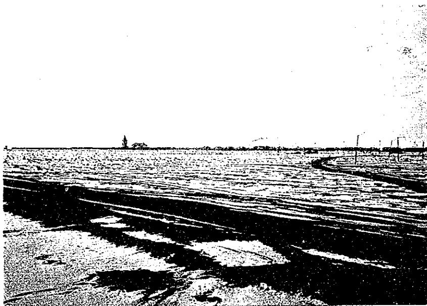
Construction Site for Transshipment Facilities
