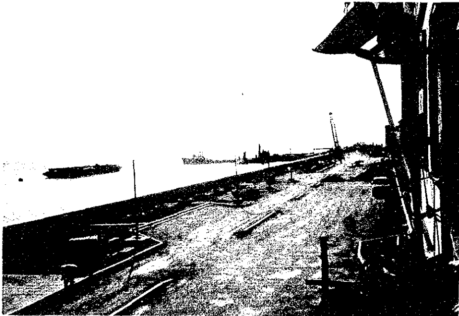
Roseau Bayfront Project - Sea wall construction
