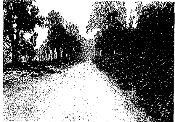
Existing road of part of Section II
