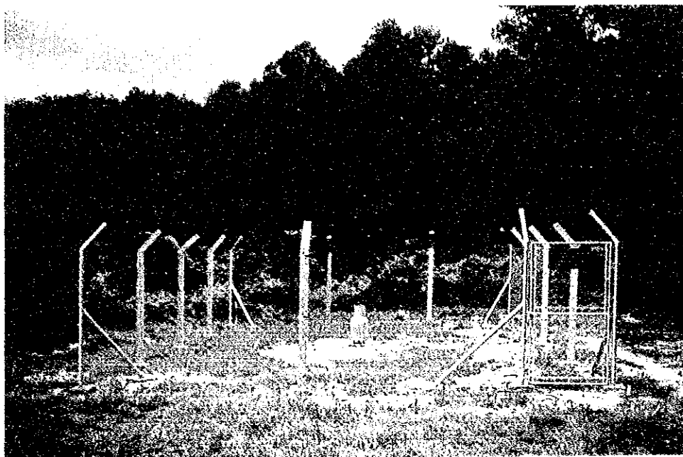
RAINFALL GAUGING STATION INSTALLED BY JICA AT EL ZAPOTAL NORTE (1993)
