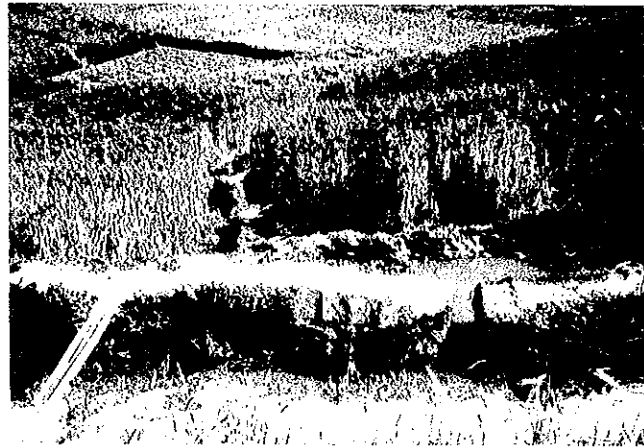
Typical water diversion to the field by cutting the shoulder of earthen canal.
