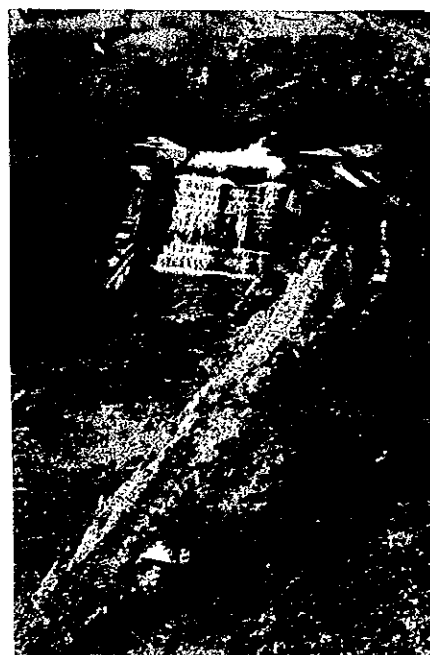
No.6 Intake (under ISP) The intake and canals were rehabilitated under ISP. Weir is made of gabion works.
