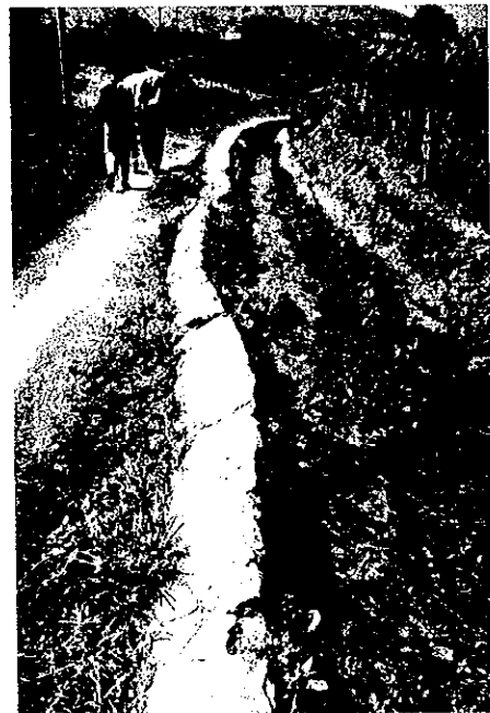
Broken canal Repair work has not been done due to shortage of budget.
