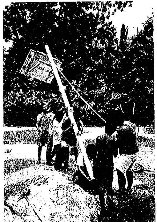
Installation of PV Module
