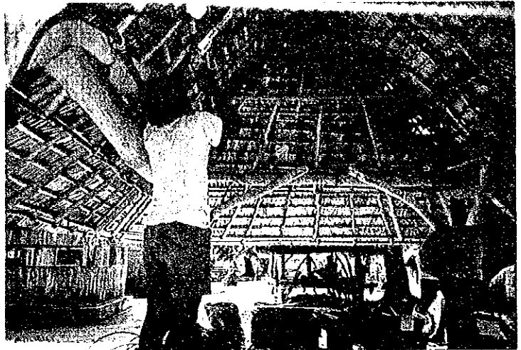
Wiring of PV system Inside of the House
