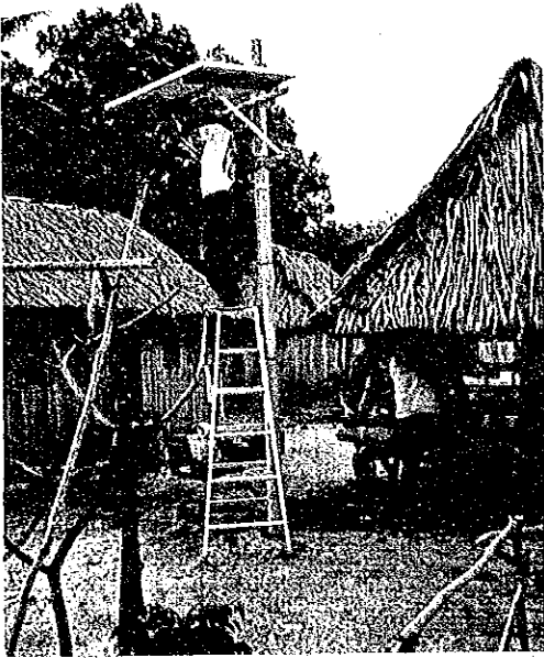
Wiring of PV system Outside of the House
