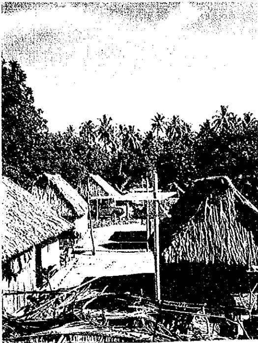
Installed PV Panels For Households
