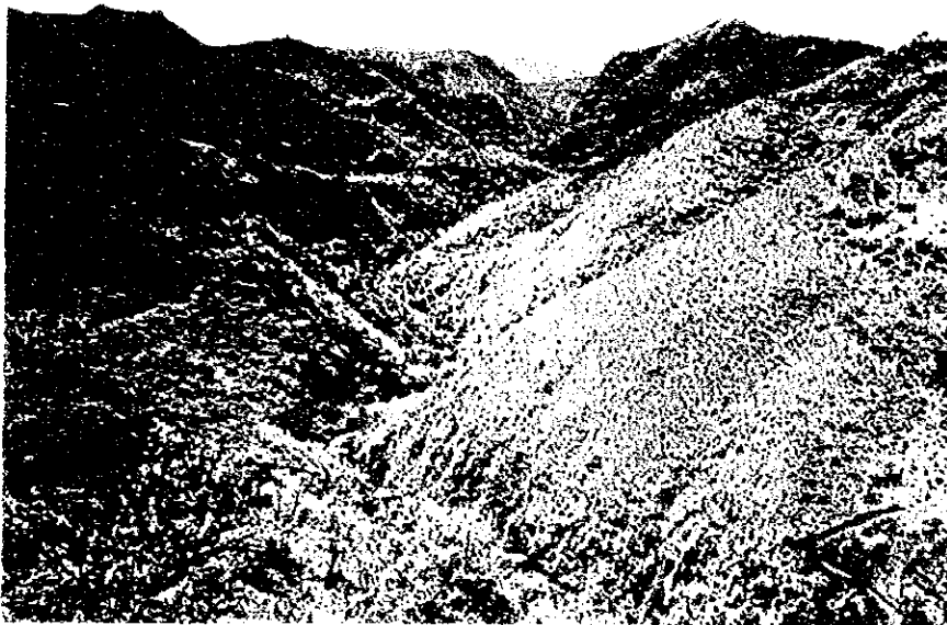
5. Downstream section of Piñán River (view from the left bank of the proposed dam)
