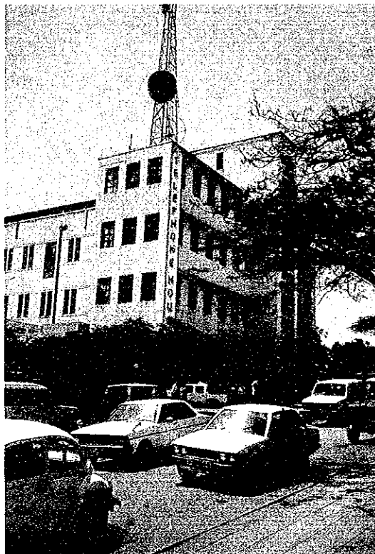
Central Exchange in KAMPALA
