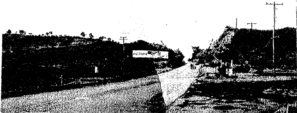
Photograph 6-6 Cutted Line at Station 22+000 km
