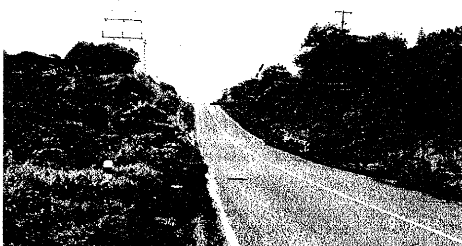
Photograph 6-3 Cutted Line at Station 8+100 km
