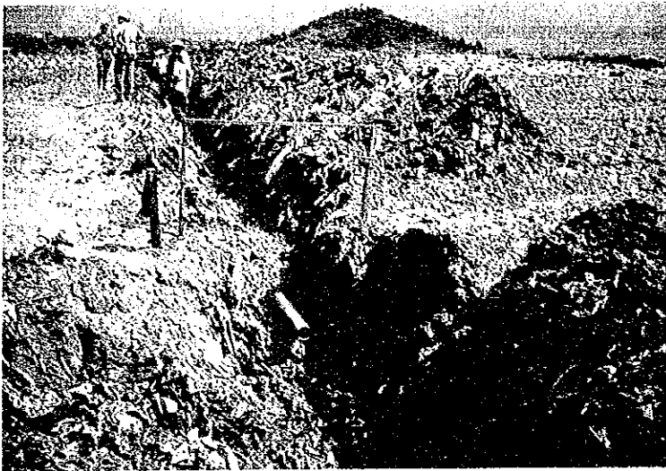
Installing horizontal gas removal facility
