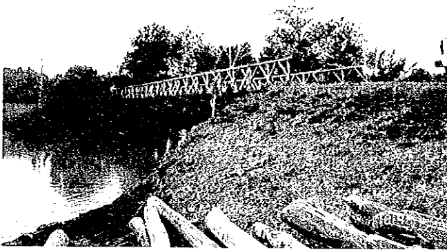
Bridge No : 10-01-09 Bridge Name: Magus
