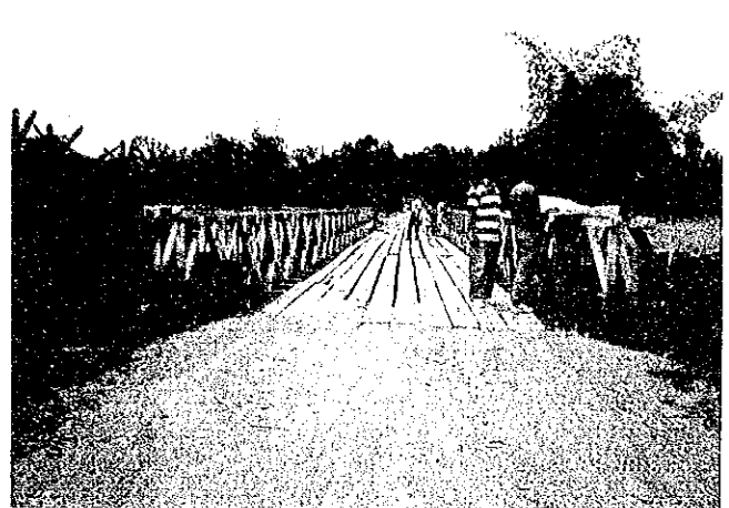
Existing Bridge : Bailey Priority : A
