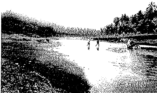
Bridge No : 10-01-10 Bridge Name: Rizal
