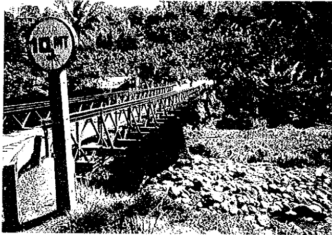
Bridge No : 10-03-03 Bridge Name: Agusan Canyon
