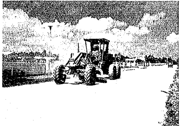
Surface grading
