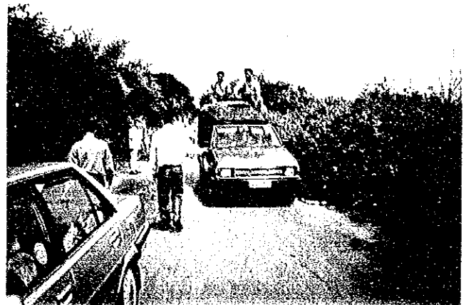
Ditto, but for RN6. Road surface is corrugated due to inundation by a flood in 1991
