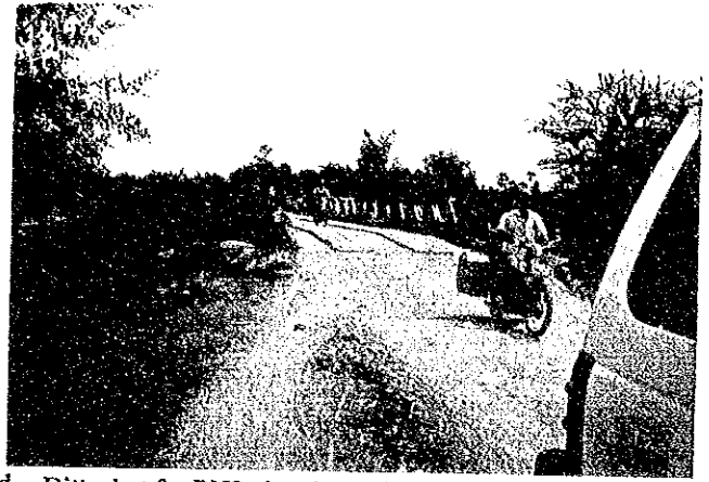
Ditto, but for RN2, deteriorated road and temporary bailey bridge
