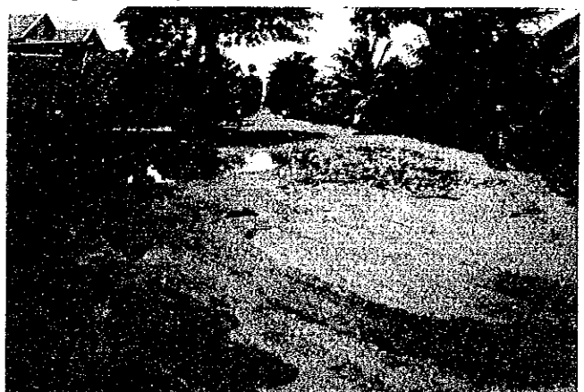
Ditto, but for RN26, condition of lateritic road near RN4 Junction.
