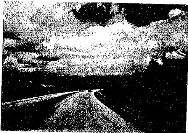
Ditto, but for RN4, 2 lanes (7m+2@1.5m) of asphaltic pavement road constructed in the mid-1960 (donated by USAID)
