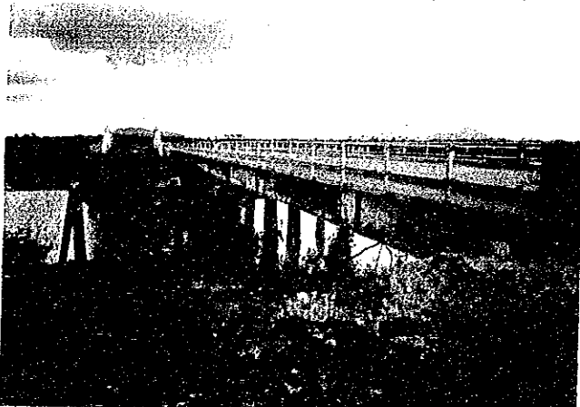
Ditto, a permanent steel girder bridge executed by RBD (Bridge Construction Company) technical assistance, materials and labour cost were provided by UNDP/AIDAB.
