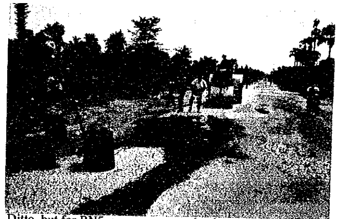
Ditto, but for RN5, emergency repair of potholes and damaged asphaltic pavement by RBD (RN5A Rehabilitation Unit), assisted by UNDP/AIDAB
