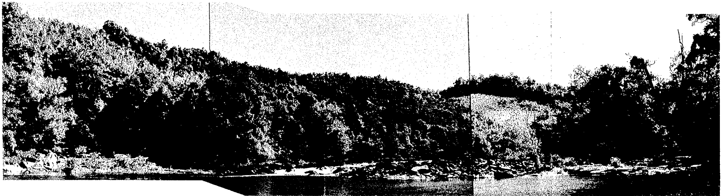
(2) View from Downstream Left Bank
