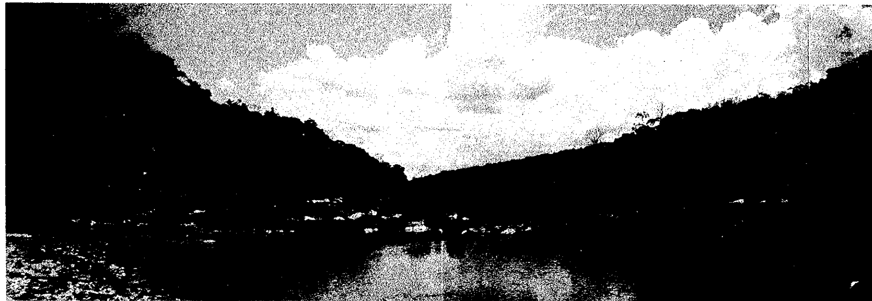
(2) View from Upstream
