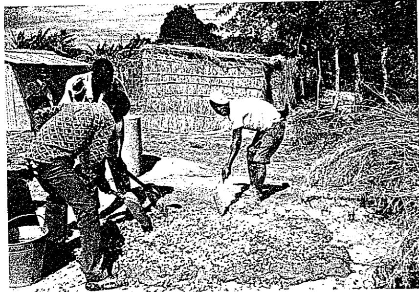
MIXING CONCRETE
