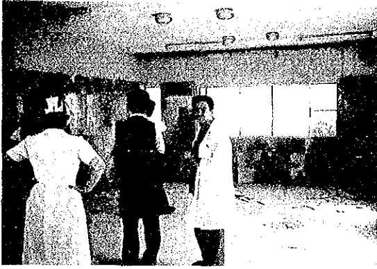
LATTAKIA AL-WATANI HOSPITAL EMERGENCY DEPARTMENT RENOVATION SITE
