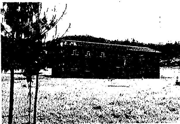
17. One of the New Building of KFC
