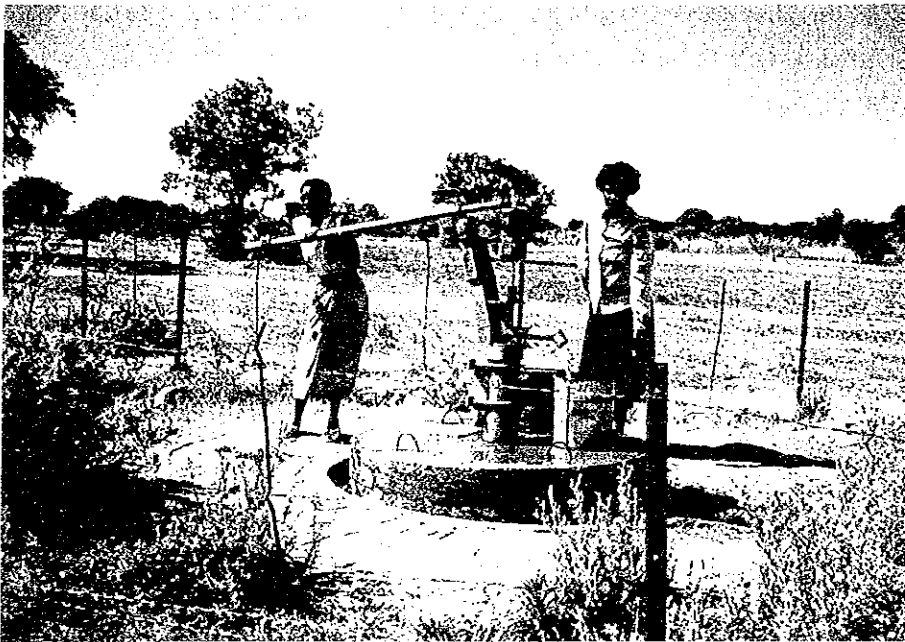
Deep Well, (Equipped with handpump)
