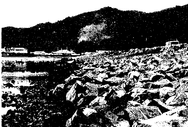
Photo 3-9 The temporary coastal protection work between Avarua and Avatiu by use of armor rocks removed from the breakwaters of Avarua Port.
