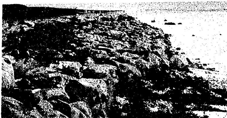
Photo 3-2 Coral fragment beach at the western end of the runway and the temporary revetment with amour rocks.
