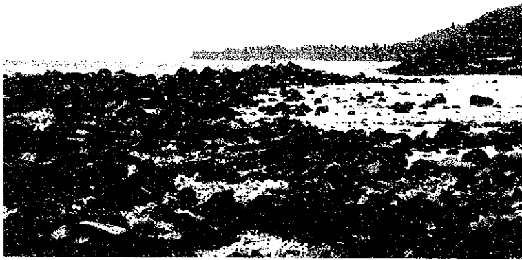
Photo 3-7 The west breakwater of Avatiu Port, abandoned incomplete.
