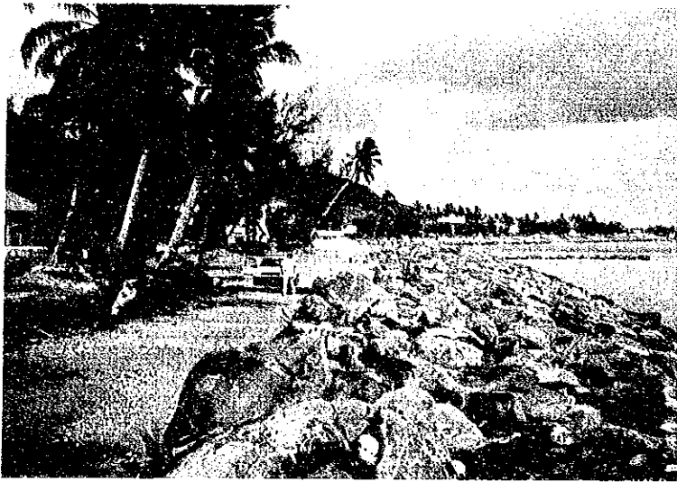
Photo 3-19 The temporary coastal protection by use of armor rocks removed from the Avarua breakwaters.
