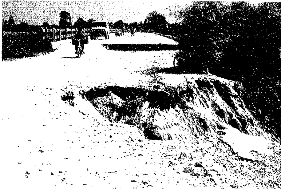
Photo 3.7 Settlement of Embankment
