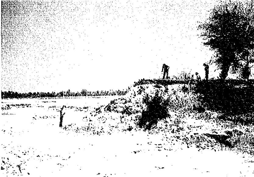
Photo 3.6 Severe Embankment Damage (Washed Away)
