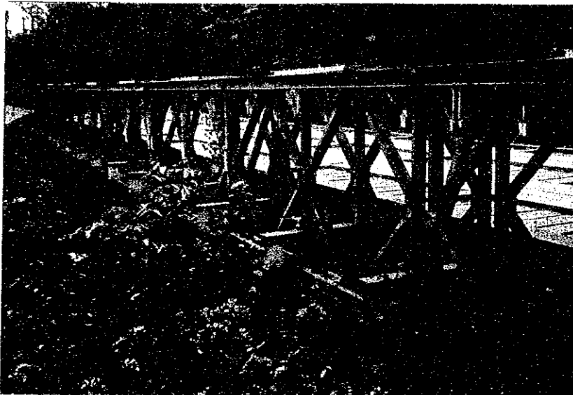
Bridge No. 1B
