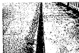
Photo - 11 Sediments on gutter
