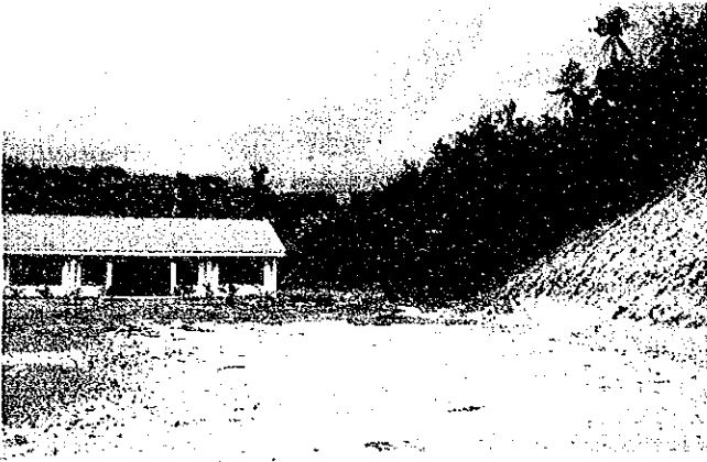
E- 49. MACO HEIGHTS CENTRAL ELEMENTARY SCHOOL
