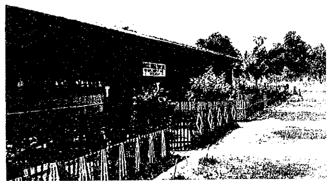
E- 72. P. ORINGO ELEMENTARY SCHOOL
