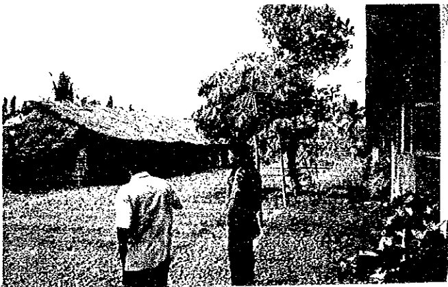
S- 93. VIGA RURAL HIGH SCHOOL
