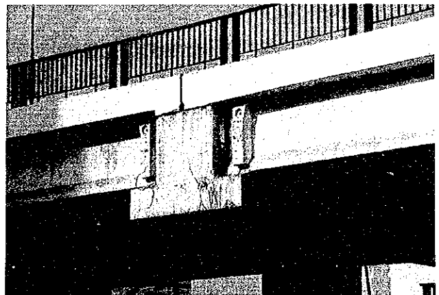
Photo 3.12.18 Failure occurred in the connection
