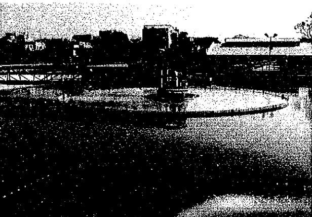
Photo 3.12.29 Rod El Farag Water Purification Plant
