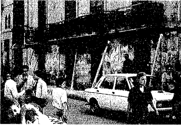
Photo 3.11.6 Temporary retrofit masonry buildings by wood supports
