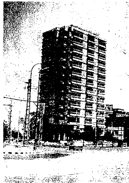
Photo 3.11.27 14-story residential building collapsed in Heliopolis prior to the earthquake (contributed by the Egyptian Gajette)
