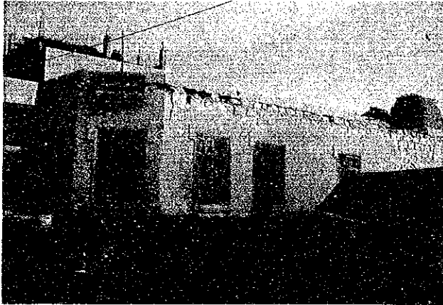
Photo 3.10.1 Damaged school (El Aiyat)
