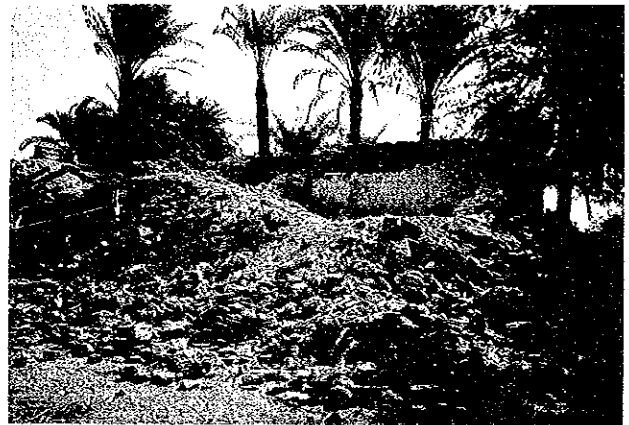
Photo 3.11.14 Totally collapsed stone masonry building
