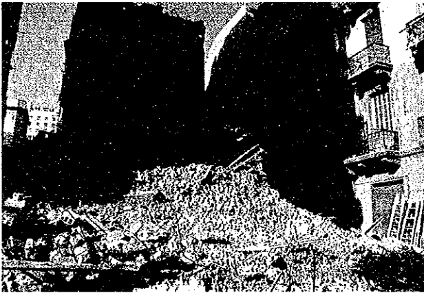
Photo 3.11.3 5-story non-reinforced masonry residential building crushed to mud (building seen in the rear is the same type building)
