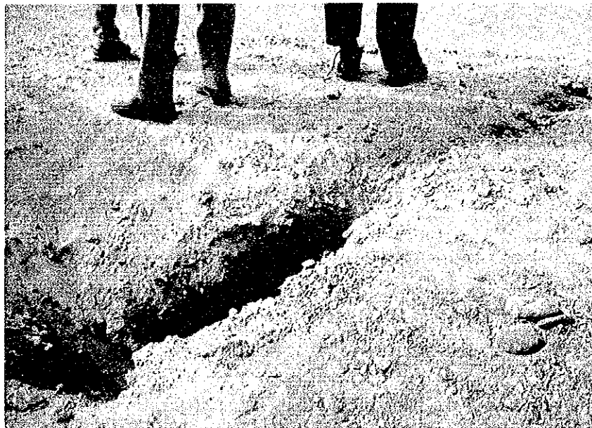
Photo 3.4.2 Ground Cracks at Dahshur No displacement observed
