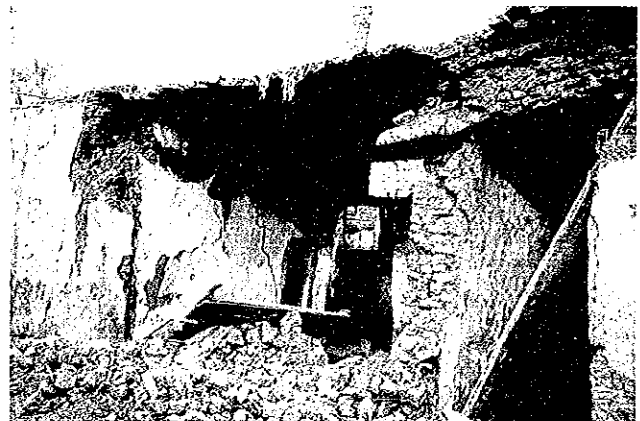
Photo 3.11.37 Damaged house in rural area (El Aiya)
