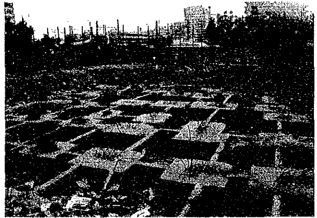
Photo 3.11.29 Foundations of 14-story residential building collapsed in Heliopolis
