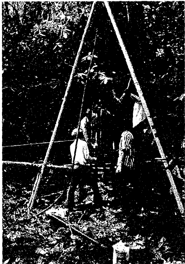
Drilling Work of Geological Investigation (KI-2)
