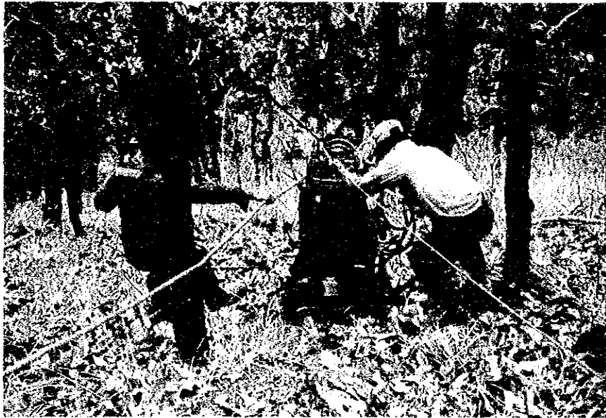
Removing the core drilling equipments along penstock route
