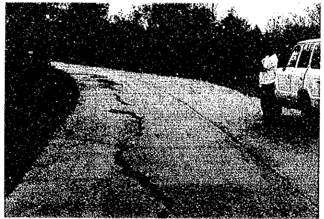
Quezon - Batangas Road, Quezon PCC pavement in bad condition
