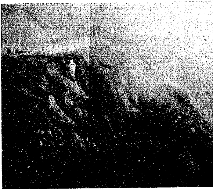
Baguio - Bontoc Road, Benguet Embankment Slope Failure
