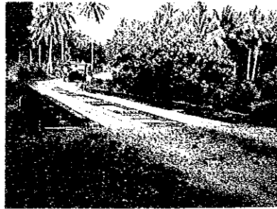
Bagong - Silang - Capalonga Road, Camarines Norte Timber Bridge
