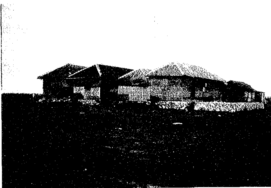
8. Open Area with No Usage
