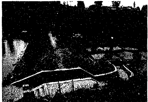
Check dams in the Study Area serve for the deposit of sediment discharged from sub-watersheds, and contribute to agricultural activities such as pisciculture and paddy farming.
