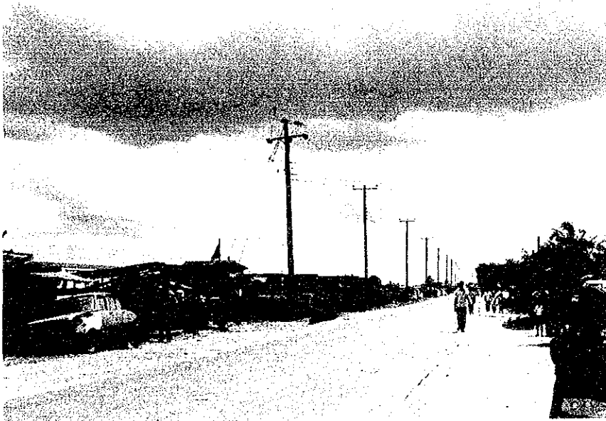
DAR ES SALAAM 11 kV Distribution Line
