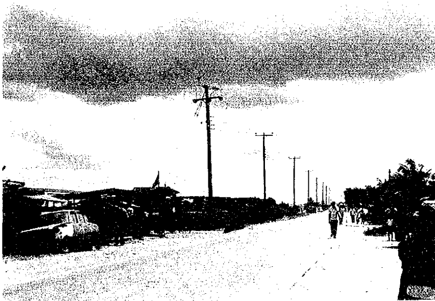
DAR ES SALAAM 11 kV Distribution Line
