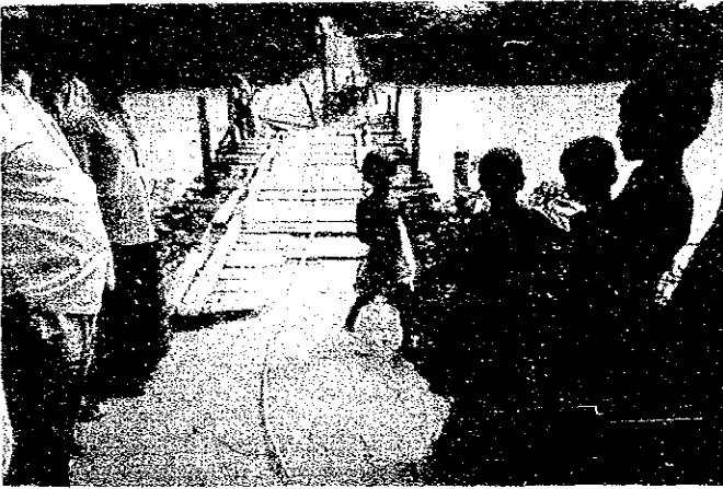
Bridge No. 15-01-01 Damaged wooden bridge unsafe for traffic.
