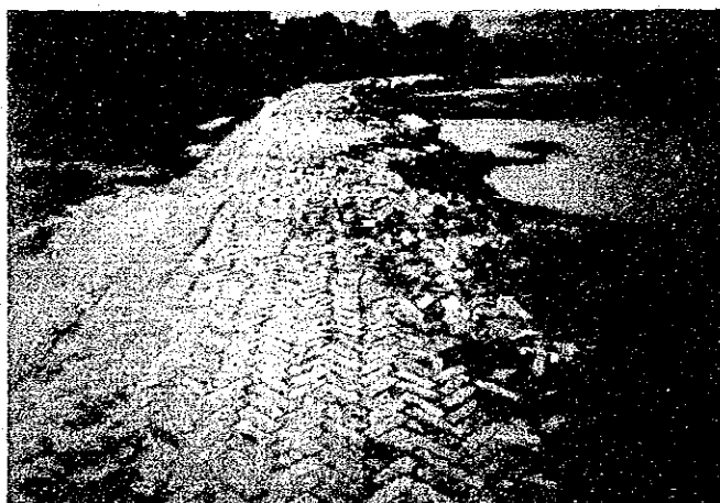
Rural Road (R1) (Parshuram, Feni) (single lane, herringbone brick pavement)
