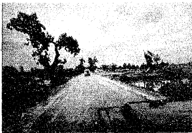
Regional Road (Feni - Parshuram road) (2 lane, bituminous surface treatment)
