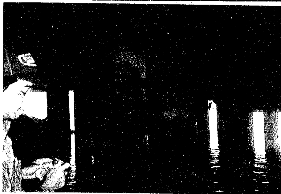
Concrete piles Additional pile
