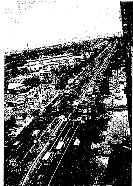
Quezon Avenue over which EXPRESSWAY ROUTE R-7 will be constructed.
