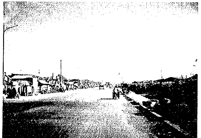
At-grade R-10 over which EXPRESSWAY ROUTE R-10 will be constructed.
