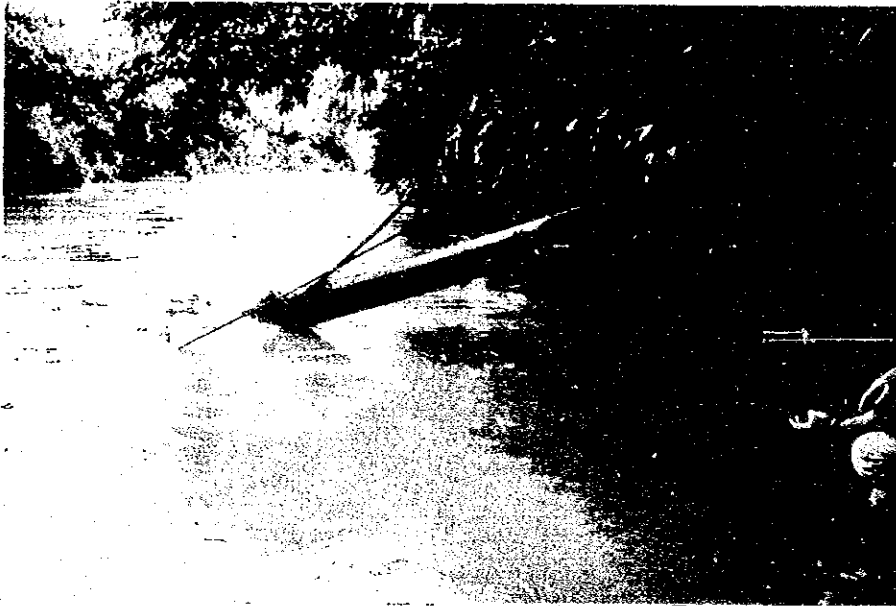
Aqueduct of the existing transmission pipeline in the Dagami system which was fallen into the Quilot River near Dagami town
