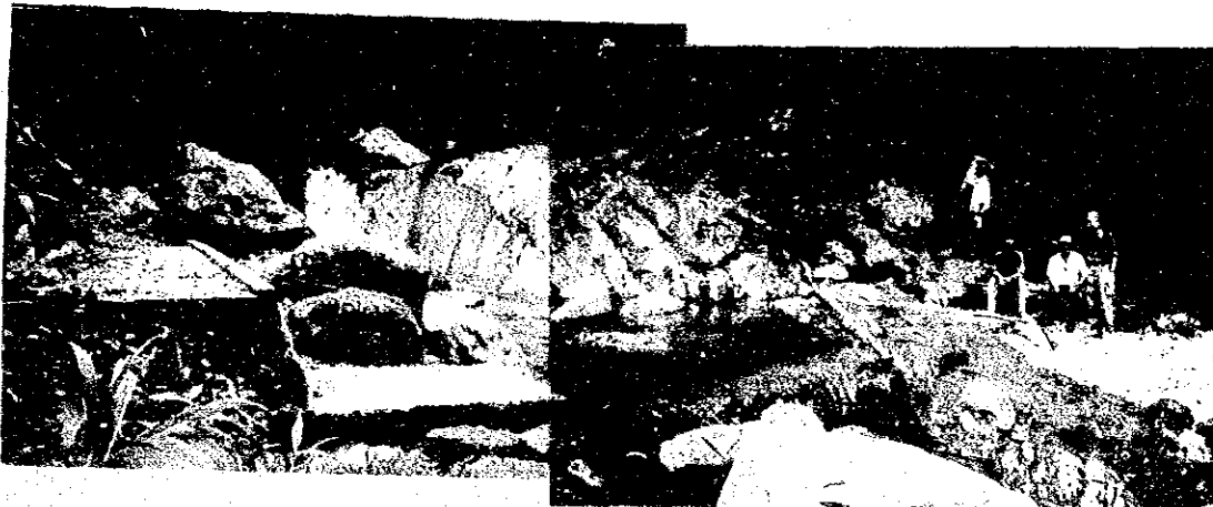
Hitognob dam (in the Dagami system) Function was recovered as nearly same condition as before the Typhoon by removal of rocks and woods flown into the dam during the Typhoon
