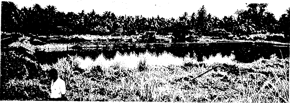
Existing slow sand filters of the Tingib treatment plant
