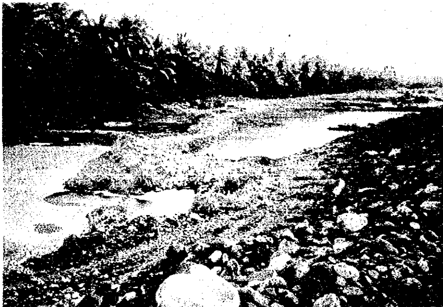
Manually dug settling ponds constructed inside of the earth dike of the Tingib treatment plant
