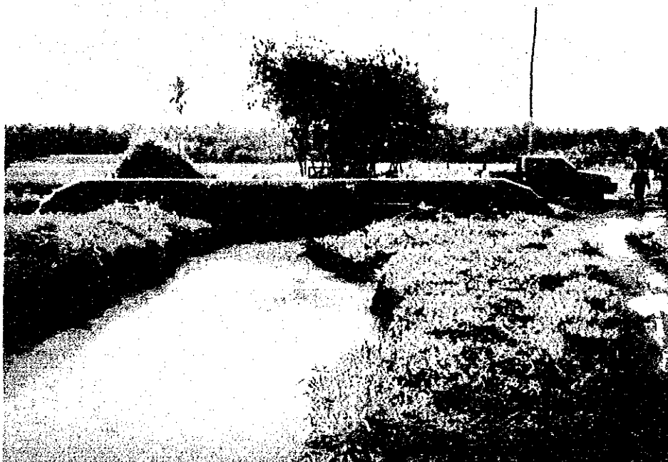
Irrigation canal crossing of the transmission line of the Tingib system
