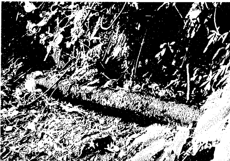
Existing raw water conveyance line (CCI) of the Dagami system
