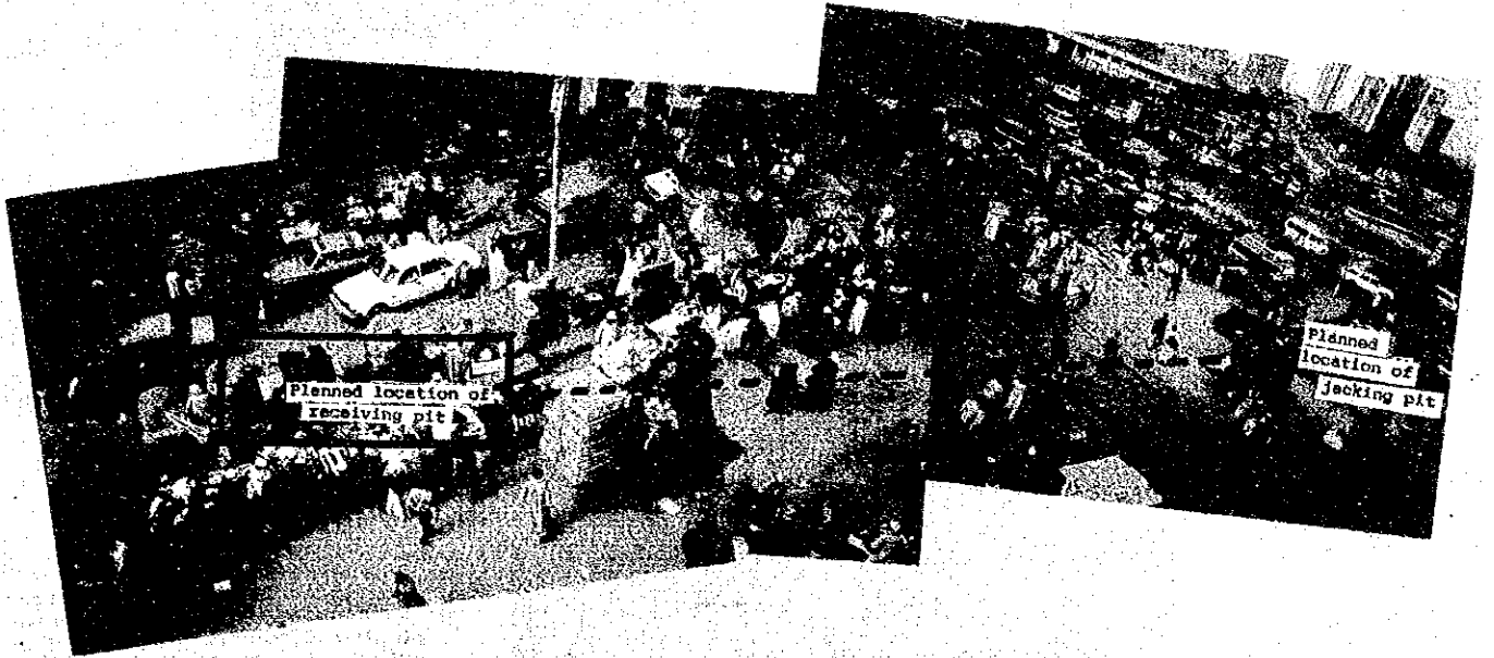
Water Supply Branch Line at the Cairo-Aswan Railway Crossing Section (Work to be constructed by Japanese side)
