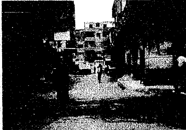
Osman Moharam Street (Sewer trunk line to be constructed by jacking method and buildings standing just besides the road.)
