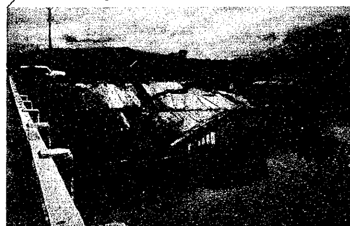
Picture shows the damaged/scoured newly constructed revetment at Malabong Bridge.
