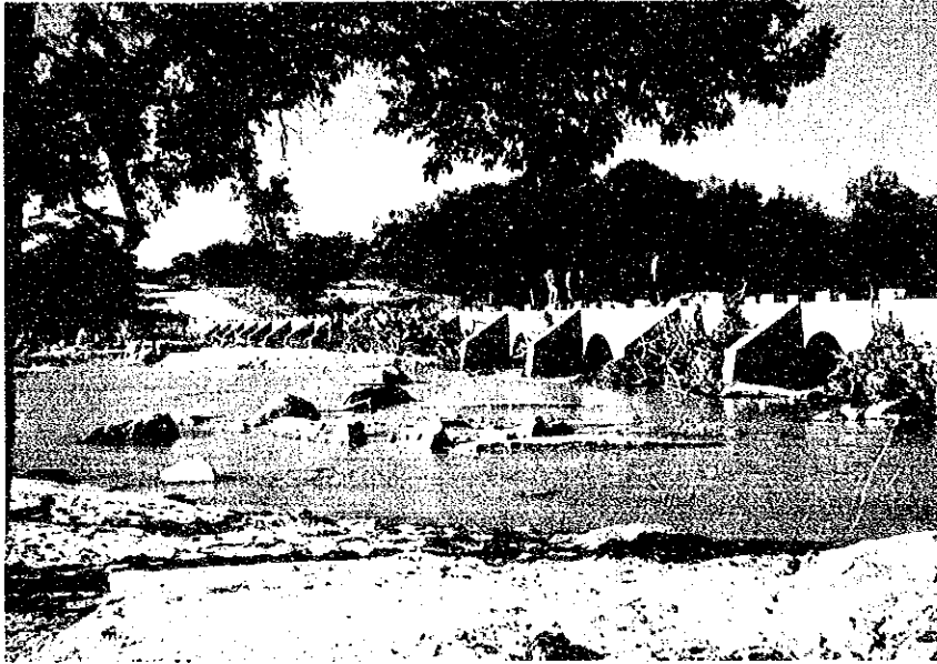
Photo-11 Devure II Bridge (Route 359)
