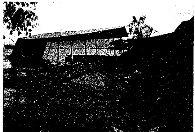
Photo 6.4 Soil Liquefaction Port Maumere The coastal zone subsided by soil liquefaction. Damaged port facility drowned about one meter in water. The part was changed from paved wharf into drowned part.
