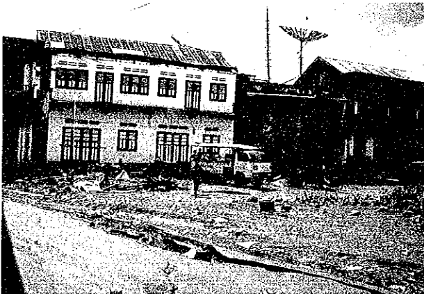
Photo 6.11 Cracks Maumere City There are many long and wide cracks in Maumere City.
