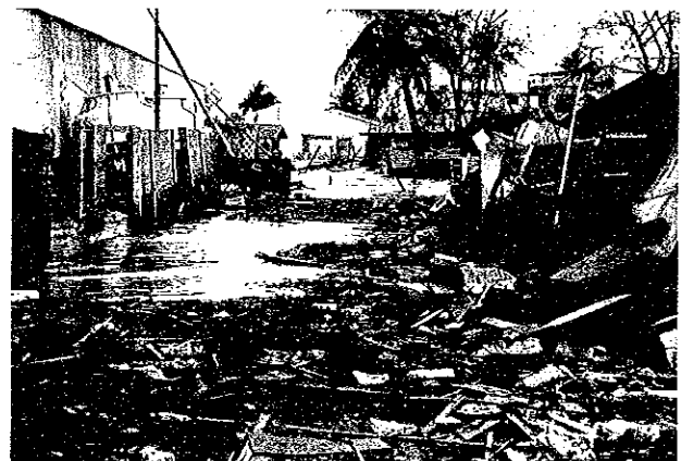
Photo 6.4 Soil Liquefaction Port Maumere The coastal zone subsided by soil liquefaction. Damaged port facility drowned about one meter in water. The part was changed from paved wharf into drowned part.
