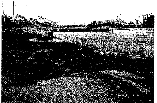
Photo 5.28 Settlement of Apron and Failure of Wall (A Ship and A Boat which were surged by the Tsunami could be seen)
