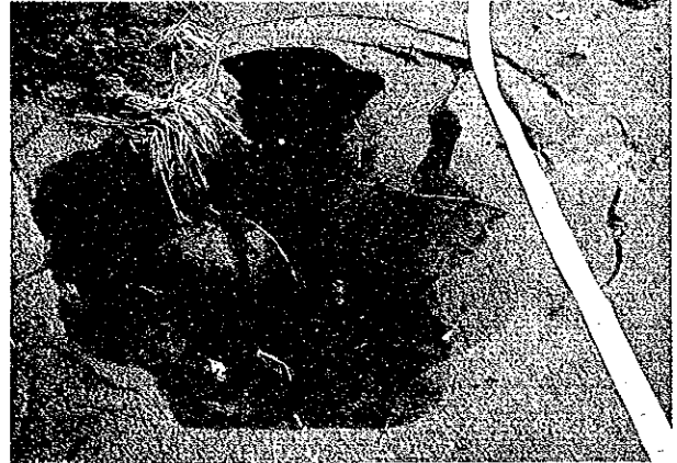
Photo 5.20 A Large Hole Caused by Soil Liquefaction
