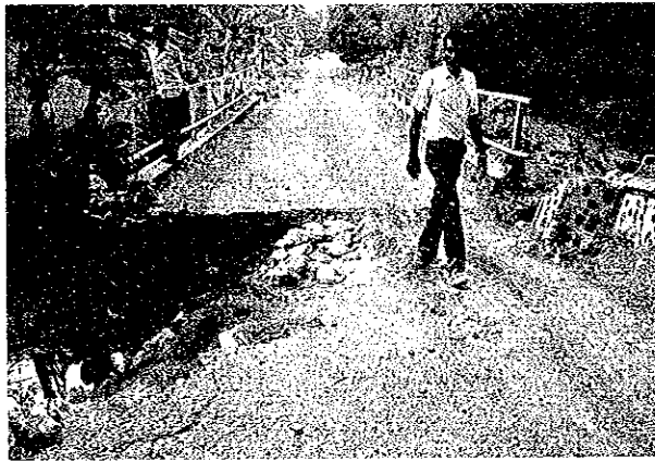
Photo 5.9 Failure of Parapet Wall and Back-Fill
