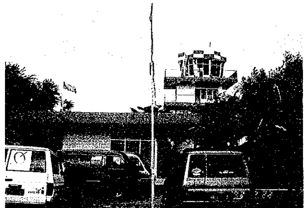
Photo 5.24 Damage of Control Tower at Maumere Airport
