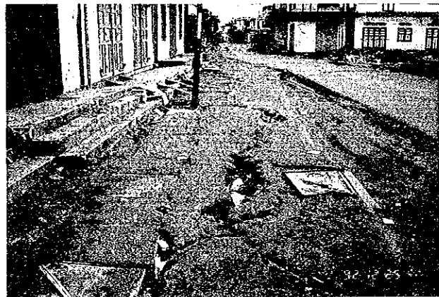
Photo 5.47 Cracks on Road Pavement along the Coast (Maumere City)
