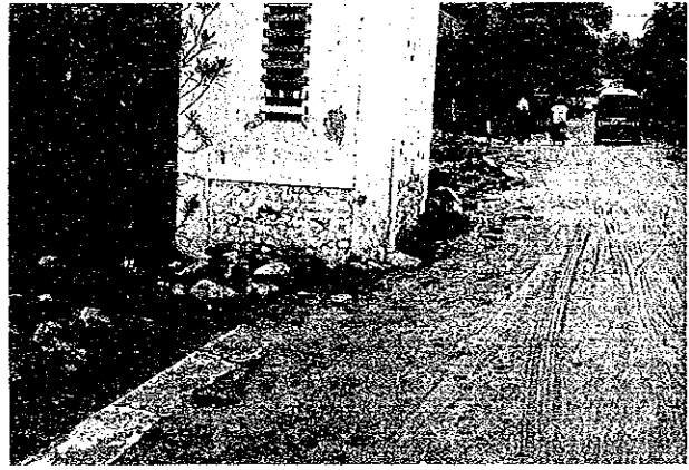
Photo 5.33 Settlement of Gate Building at Maumere Port
