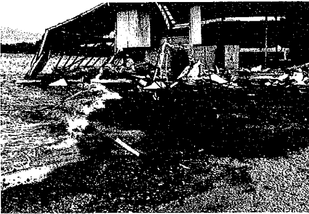
Photo 5.44 Settlement of Storage Yard along the Coast
