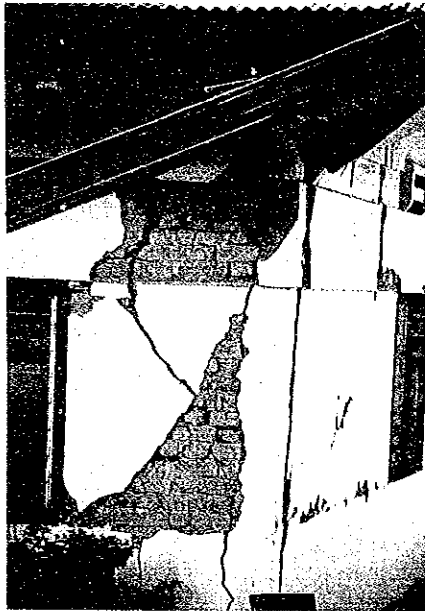
Photo 4.9 Adobe One Storey House, Severe Damage
