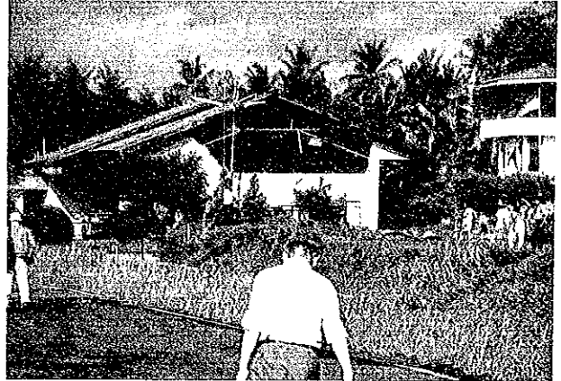
Photo 4.2 Masonry Building in Ende Airport, Falling Down of Side Upper Wall
