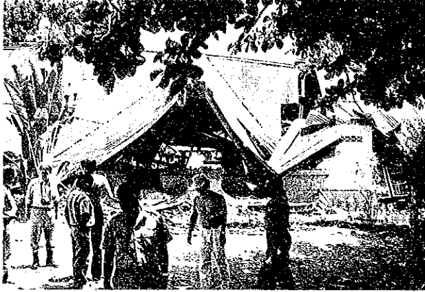
Photo 4.24 Religious House; Collapsed, Ende City
