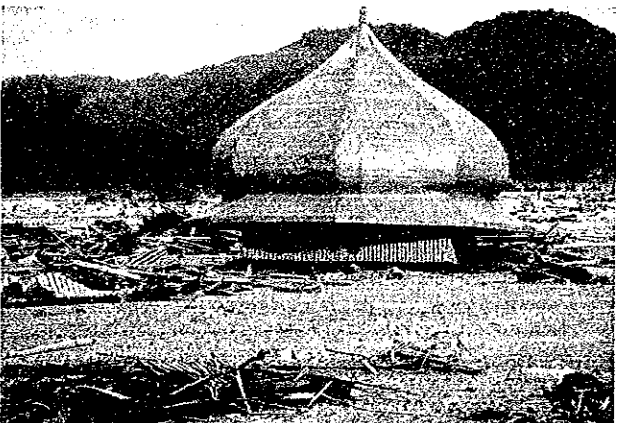
Photo 4.28 Only Roofing of Mosque was Remaining in Babi Island
