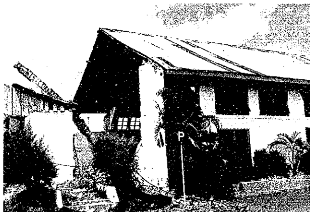
Photo 4.17 Ende Assembly Hall; Collapse of Side Wall
