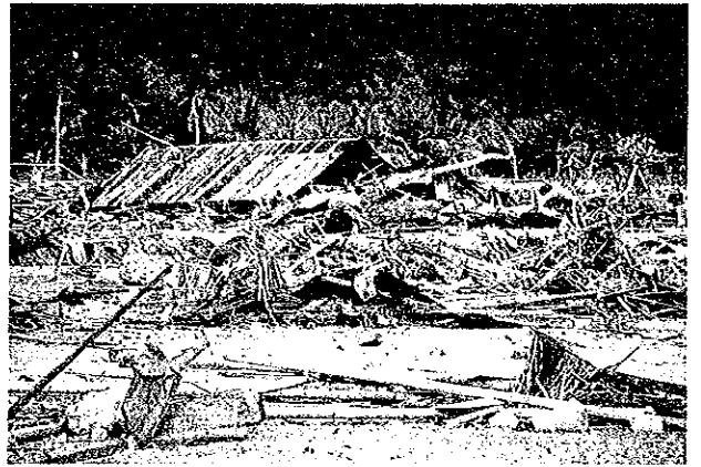
Photo 4.27 Collapsed House Due to Tsunami in Babi Island 30 km from Maumere City
