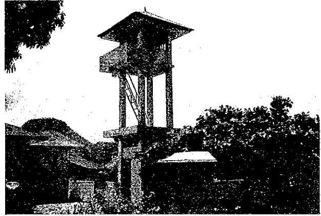
Photo 4.21 Reinforced Concrete Tower Building; Slight Damage
