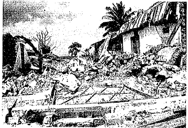
Photo 4.36 Collapsed Masonry House in Maumere City
