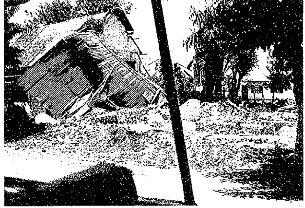
Photo 4.19 Typical Damage Pattern of Masonry Wall Building; Perfect Collapse
