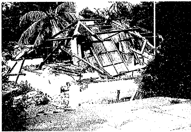
Photo 4.43 Typical Collapse Pattern of Masonry House; Many of Masonry Houses were Collapsed Like This Pattern in Maumere City
