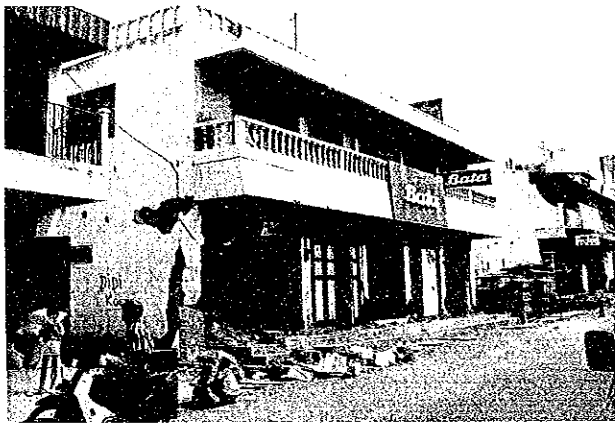
Photo 4.50-1 Severely Damaged Reinforced Concrete masonry Wall Building
