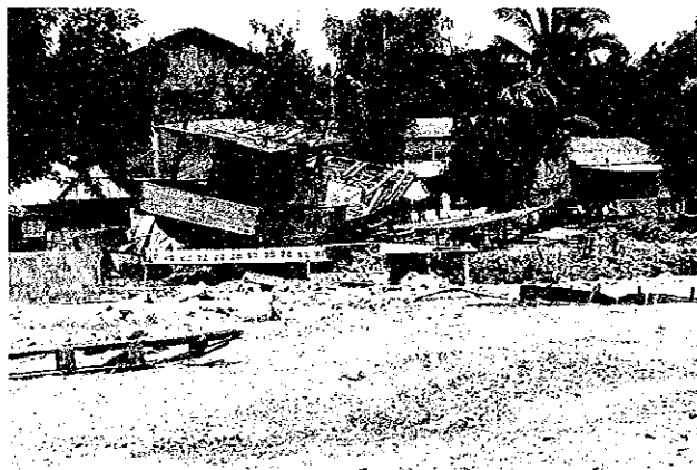
Photo 4.33 Damage of Maumere Seaport by Tsunami
