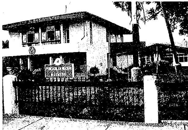
Photo 4.45 Two Storey Reinforced Concrete Masonry Building; Severe Damage, Business Work was Done in Temporary Facilitated Sheet Tent
