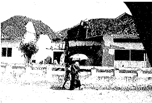
Photo 4.10 Branch Office of Ministry of Public Works, Partially Collapsed
