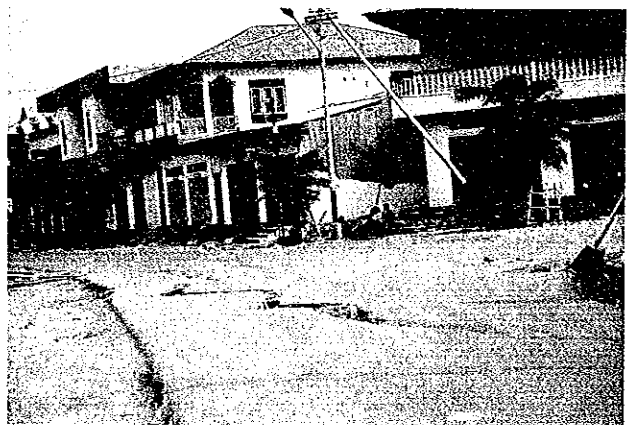
Photo 4.54-1 Damage of Road Observed in maumere City; Only This Area Was Damaged
