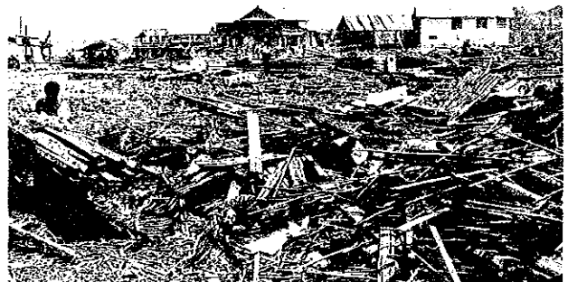
Photo 4.34 Perfect Collapse of Wulin Town by Tsunami 3 km West of Maumere
