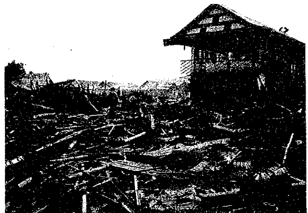
Photo 3.5 Tsunami Disaster at Wuring Area (Center of the village)
