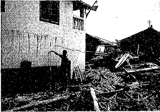
Photo 3.6 Inundation Height at Wuring Area
