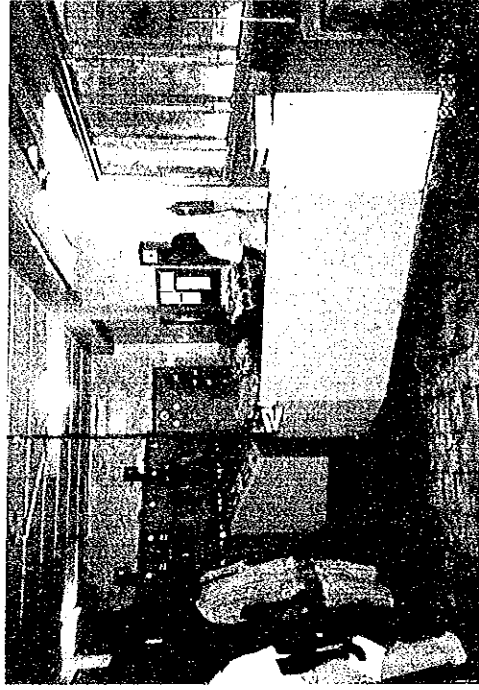
Control Room in the Existing Power House (The three desk-type control panels for MAN Generators located on the right side of the room are currently not being used. As with the circuit breakers for transmission and distribution of electricity, it is planned for these to be rehabilitate by the EEC and EIB.)
