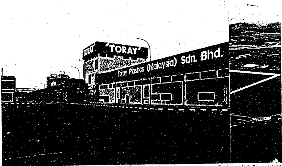
The site earmarked for the proposed plant.
