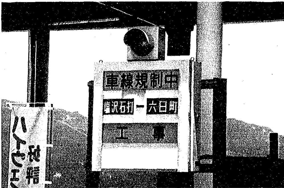
Close-up View of A Toll Gate CMS
