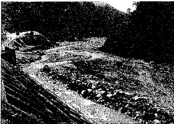
Photo. 6.2.8 Aggradation of Khami Khola near the confluence with Rapti River
