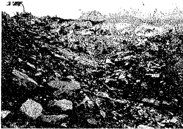
Photo. 6.3.1 View of Upper Jurikhet Landslide (so called as Small Landslide)
