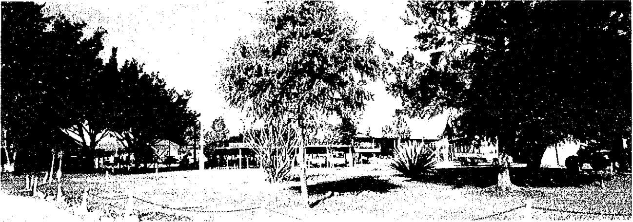
Central Workshops - Overview -
