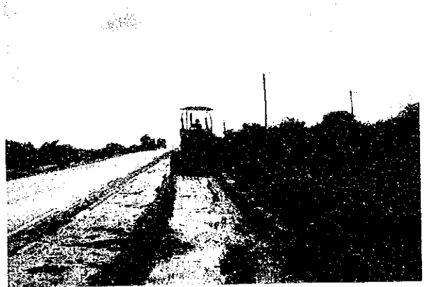
Grading road side
