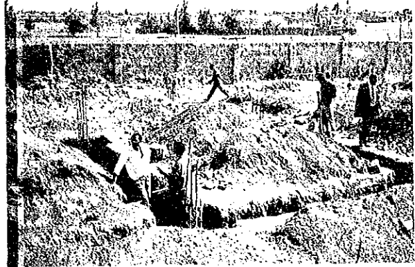
RUIRU Construction site
