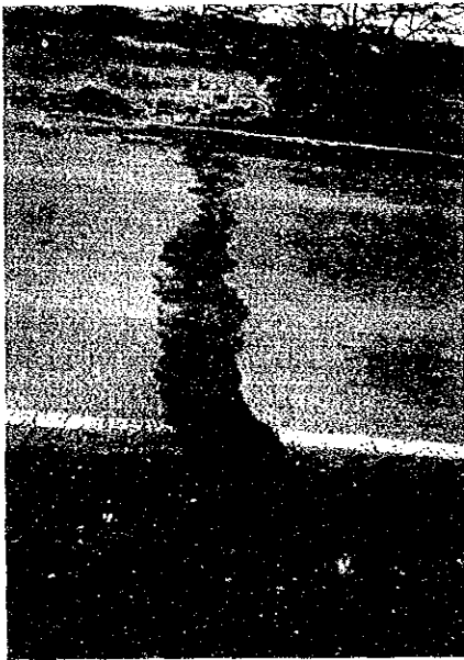
Patching on crack
