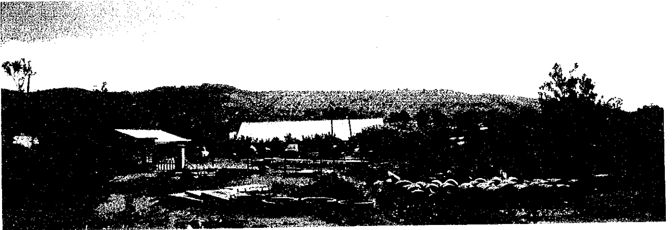
MACHAKOS Bridge Unit - Overview -
